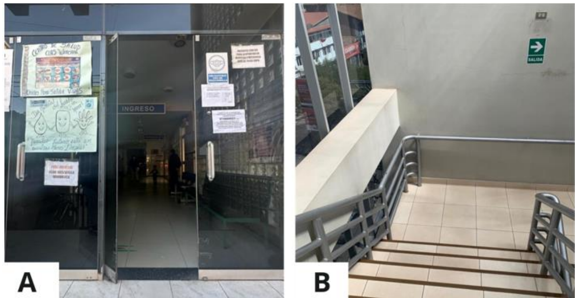
Figure 04. The principal entrance to the Peruvian Health Center in Cusco (A) . The principal stairs lead to all the building floors (B) .
